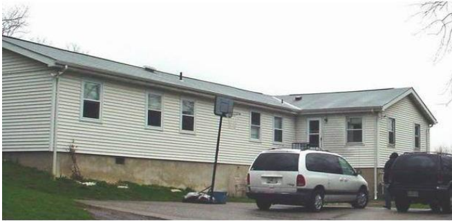
GUIDE Catonsville Structured Shelter
